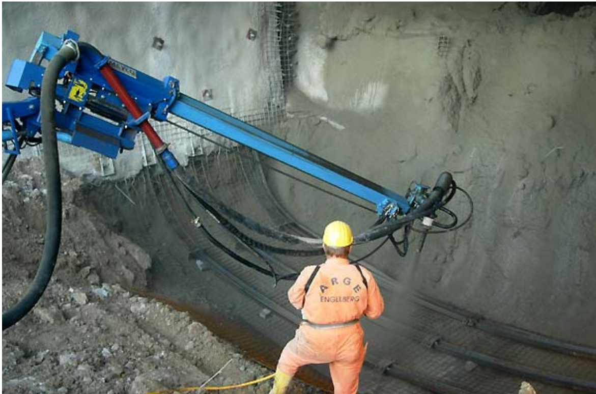
Figure 1: Shotcrete robot in action. (Source: Meyco)
