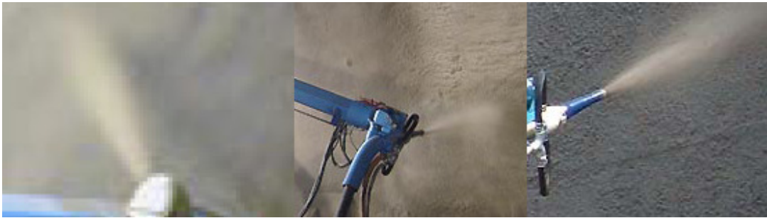
Figure 25: Real shotcrete rays. (Source: Meyco)
